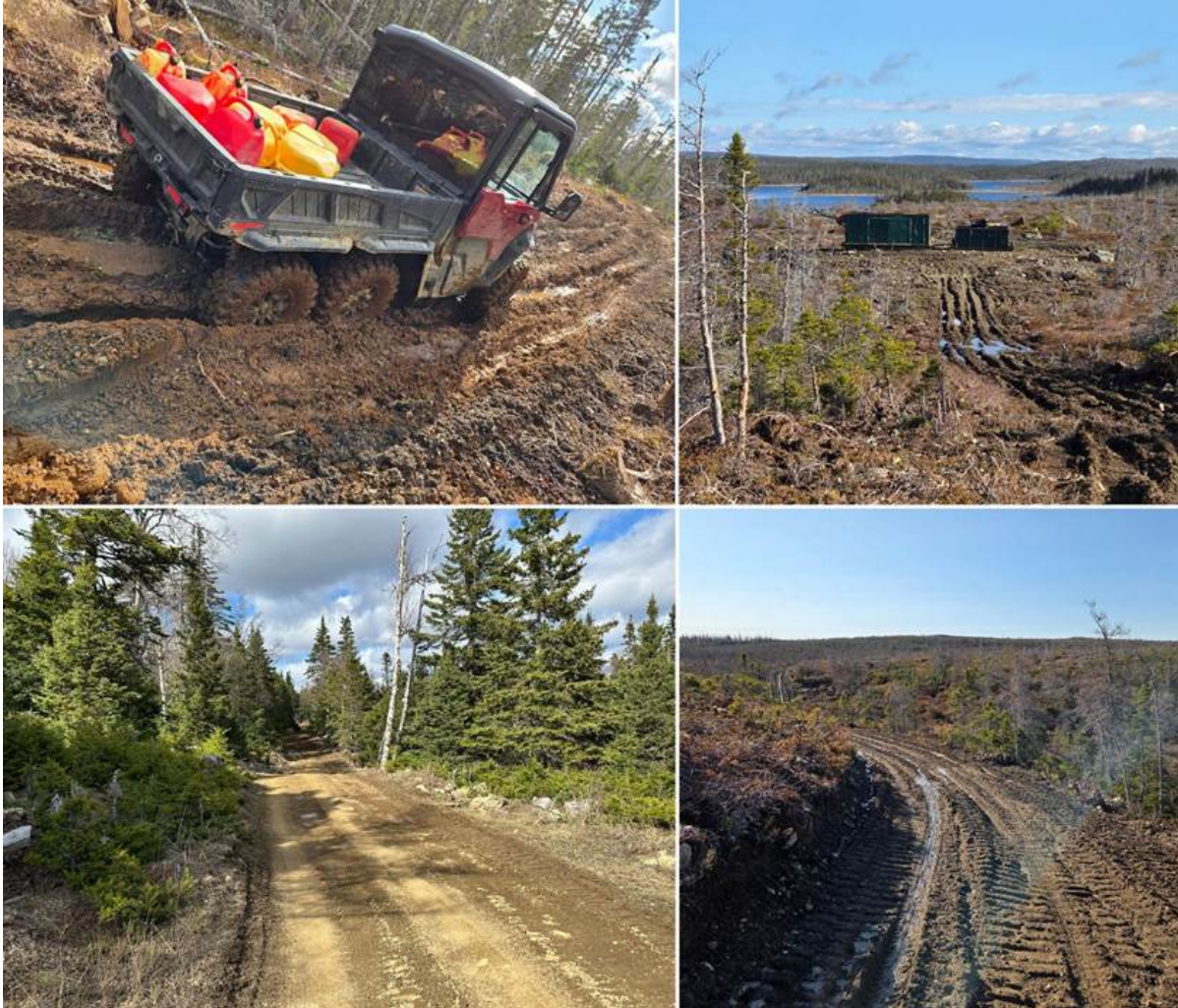
Figure 1: Images from the Phase 2 Drilling program start-up at the Atlantic Nickel Project, showing the drill being set up at a new drill site location near the RPM Zone for step-out hole drilling.
