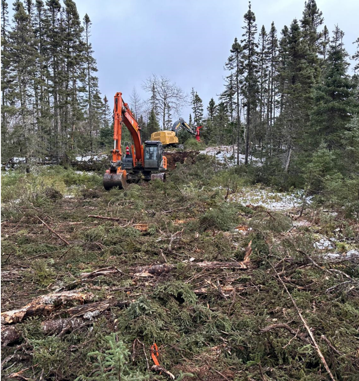
Figure 2: RPM Zone Southern Access Trail (Started January 2025), providing efficient and direct access for Phase 2 drilling program.
