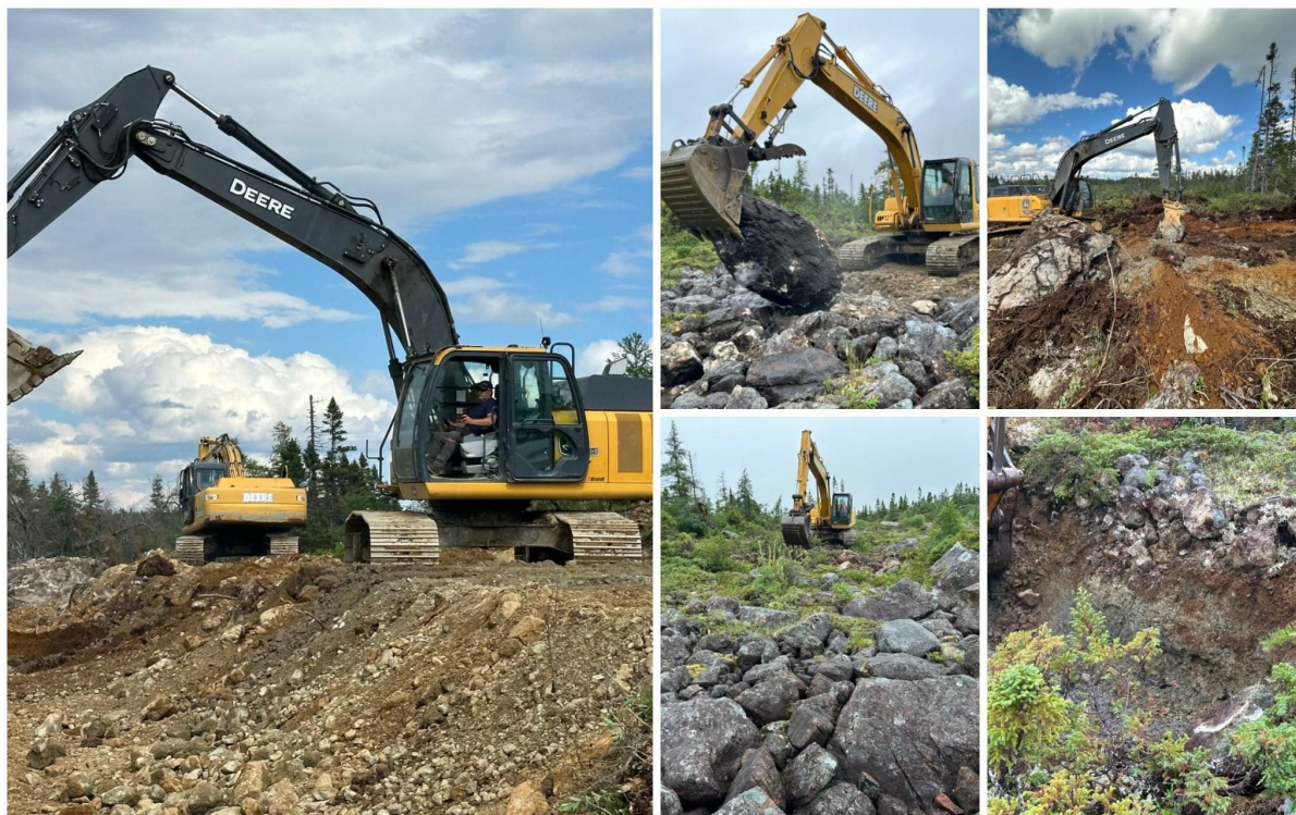
Figure 4: Excavator ditching and clearing along the exploration access road at Pipestone XL, with overburden and boulders pushed aside to open drainage across boggy ground (Fall 2026).
