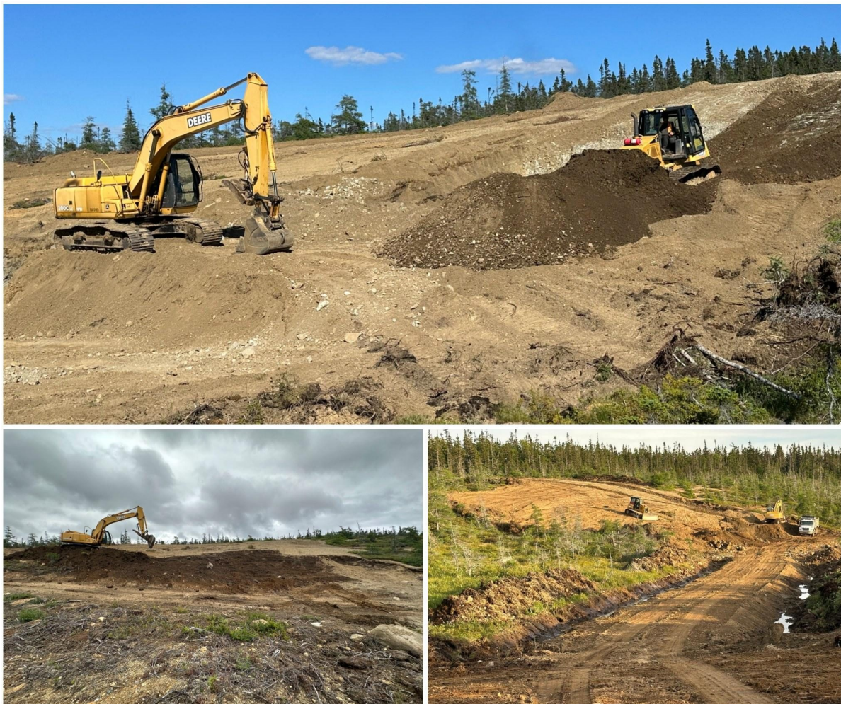
Figure 5: Stripping overburden to decomposed bedrock at the permitted pit north of the RPM Zone, which supplies fill for the exploration access road and exposes bedrock that can be sampled (Fall 2026).
