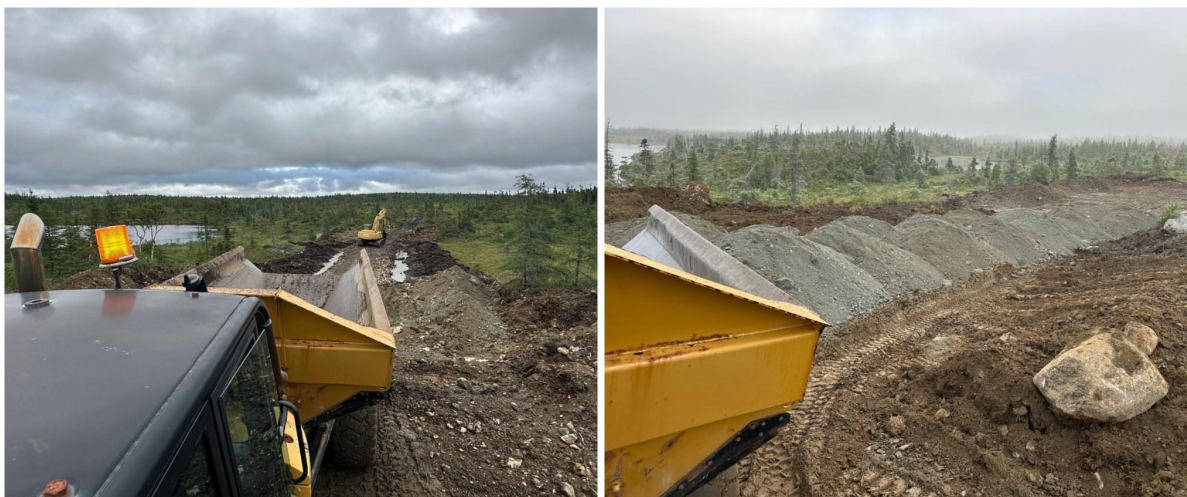
Figure 6: Dump truck hauling fill from the permitted pit north of the RPM Zone along the exploration access road, Pipestone XL Project (Fall 2026).
